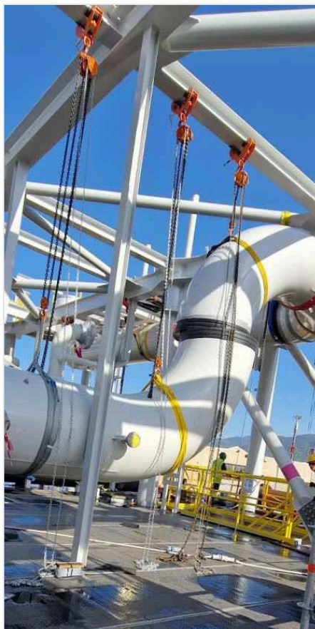
Detail: fit-up, pipe 42"
