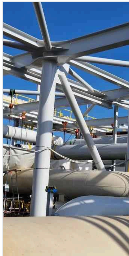
Overview: second-floor piping during installation
